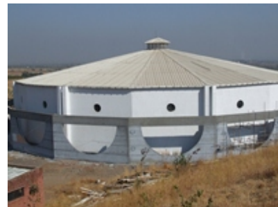
Winery under completion
